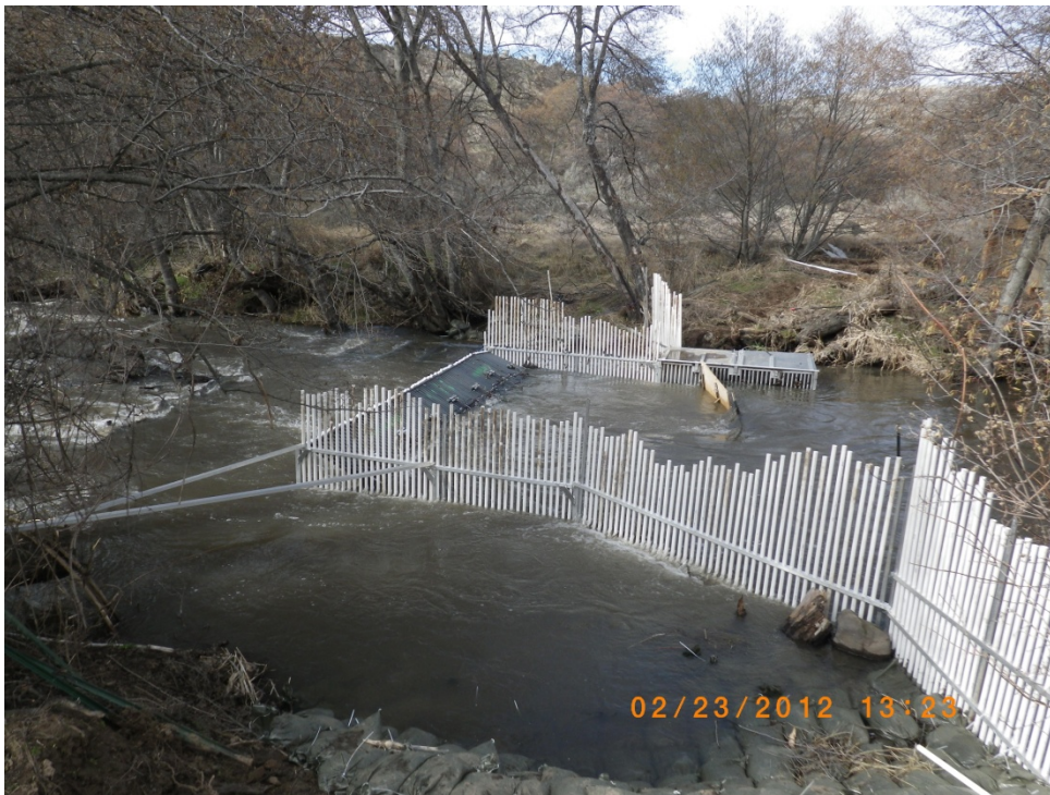
Figure 2. Resistance panel weir trap installed in its new location in Fifteenmile Creek for the 2011-2012 season. The new site is approximately 100m downstream of the previous season's weir site. Top image shows the weir at winter base flow, as viewed from upstream; bottom image shows the weir at moderate flow, as viewed from the bank adjacent to the trap.
